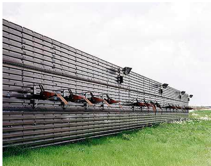
Aircraft Decontamination Building on site (image courtesy of English Heritage Assets)
