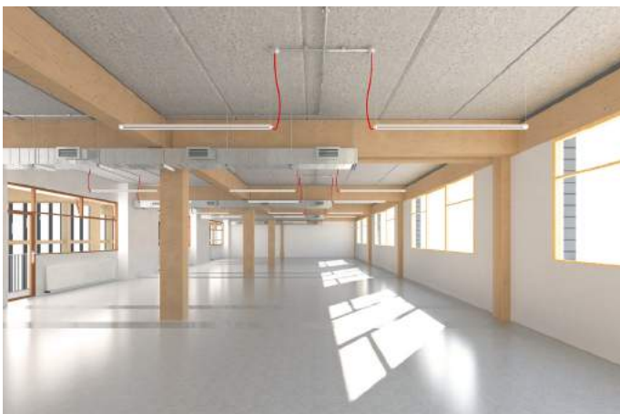
Glulam and PCC - Air Handling Unit
