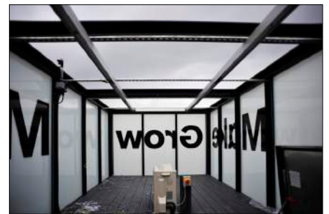
Fitout and install lightbox glazing + signage
