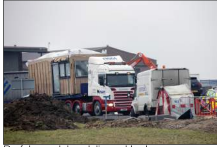
Prefab modules delivered by lorry
