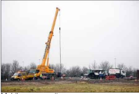
Mobile crane onsite
