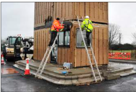
Weatherproof between modules
