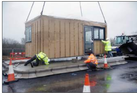
Locate onto capped-off services
