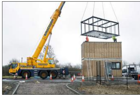
Locate onto capped-off services
