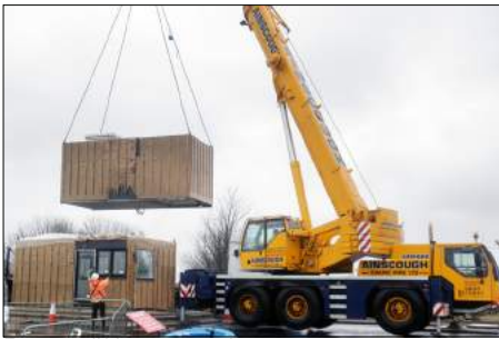
Repeat lifting operations
