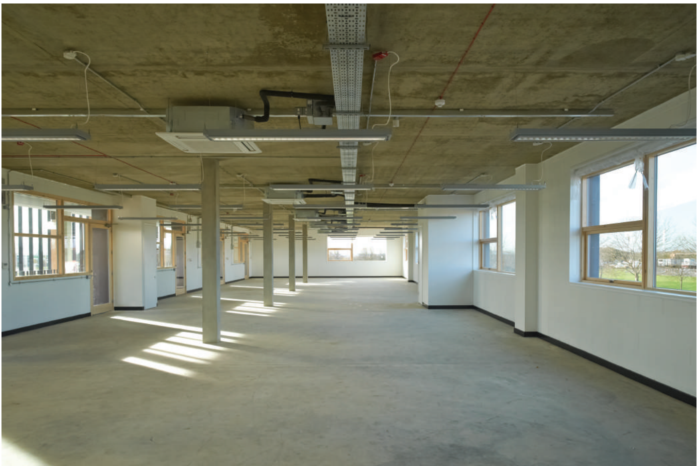
As built concrete flat slab - Natural ventilation assisted by VRF units
