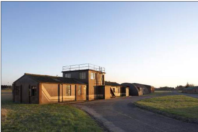
Grade II Listed Watch Office + Operations Room
