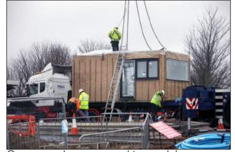
Corner anchors secured to module
