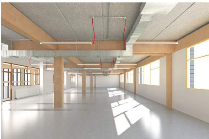
Glulam and PCC - VRF Units
